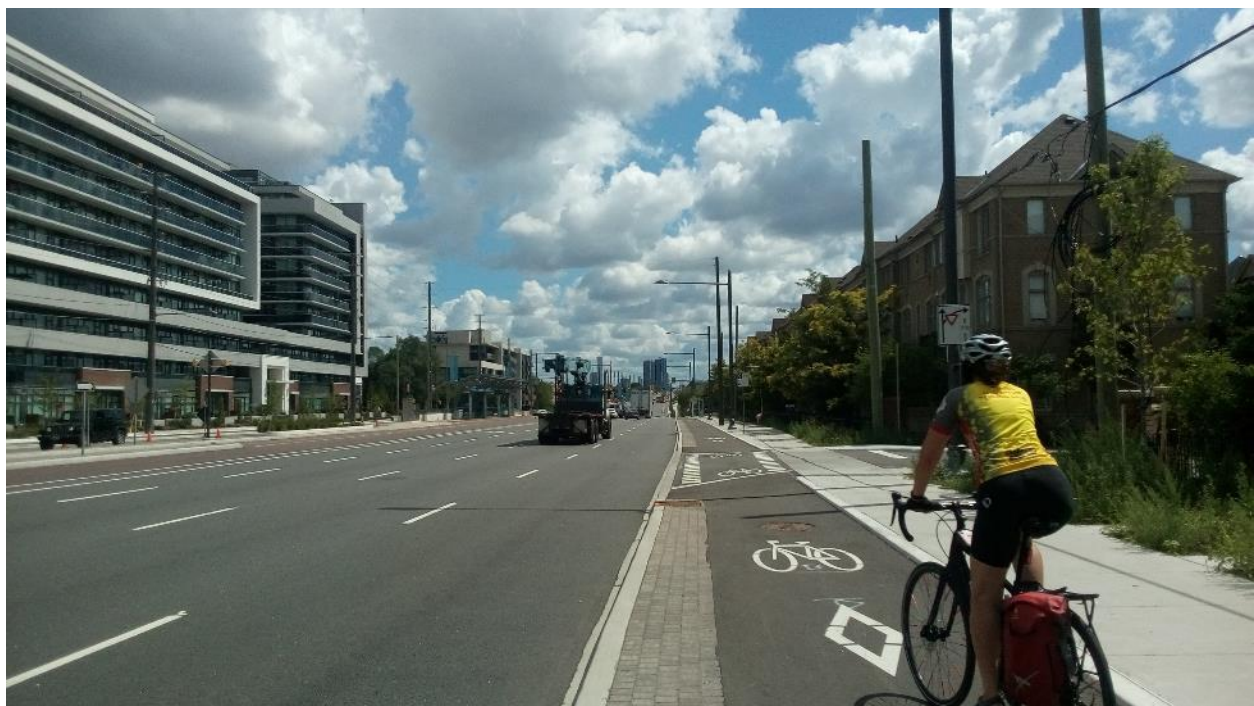
Raised cycle track, Hwy #7 in Vaughan. Note white paint delineates driveway, not use of a concrete curb. Photo credit: Barry Lavallee
