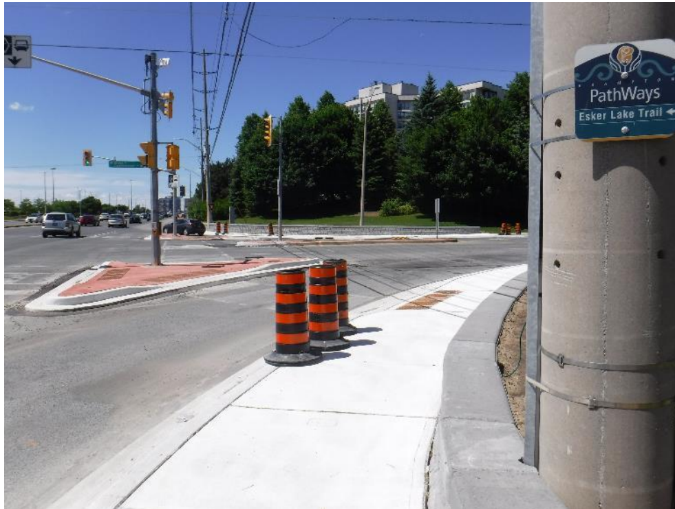
Queen Street new 'porkchop' at Laurelcrest, where Esker Lake Trail crosses Queen. Photo credit: Dayle Laing
